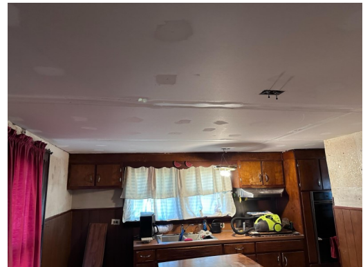
Jack and Steve hung drywall on the kitchen ceiling of this house.
